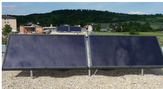
Installation on the roof – horizontal
