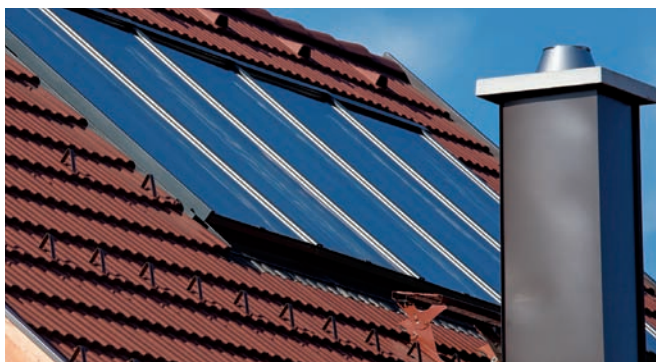
Installation within the roof
